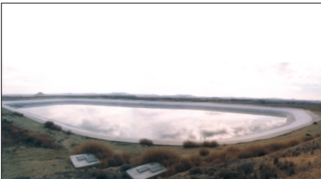
Recycled water storage lagoon
